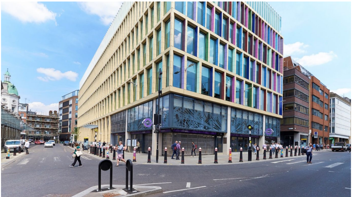
Figure 2220: The entrance to the new Farringdon entrance to the Elizabeth line on the Corner of Long Lane and Lindsey Street. ©Clive Totman
